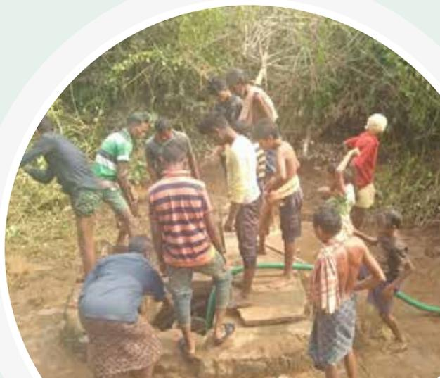
During the water quality management project rolled out by Gram Vikas, people brought forth the issue of water wastage due to leaking taps. If there are leaks in almost every tap from the 30 households, it adds up to a huge wastage. "As we were undertaking the community - based repairing of the water supply system, we thought that we could also repair the household taps. We took the help of a plumber from Gram Vikas to fix the taps and now none of the taps in the village leak," says Gandhi.
