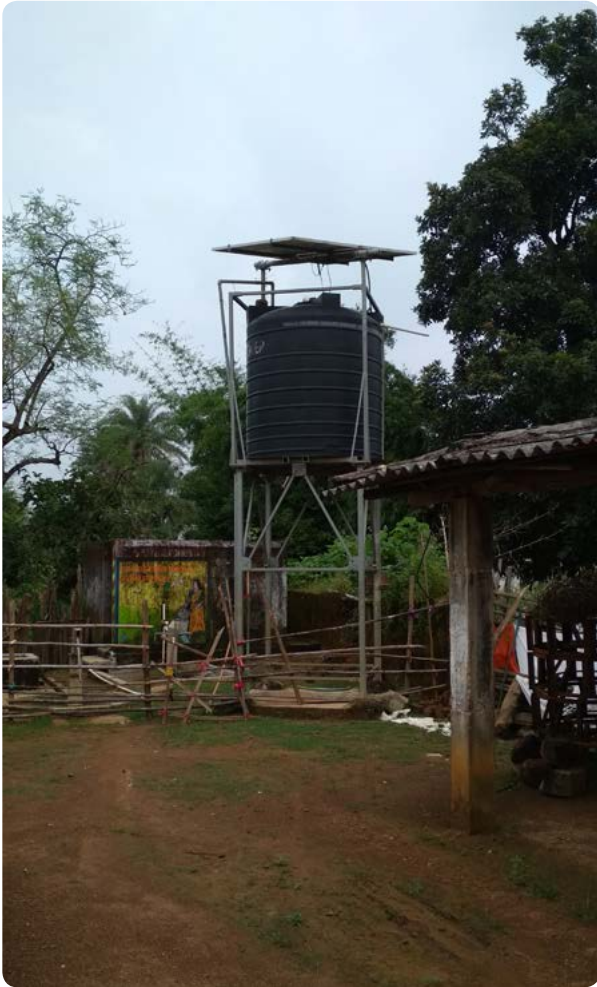
Overhead water storage tank in Sivani Panchayat, Kanker, Chhattisgarh
