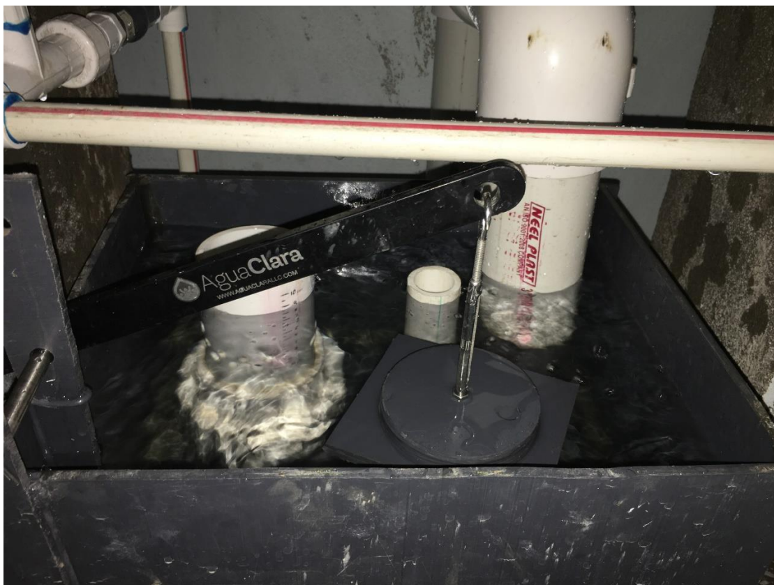
Figure 11: Entrance tank as installed in Patimul. In the back row, from right to left are the LFOM, overflow weir, and submerged inlet pipe. In the front is the dosing arm with float attached via turnbuckle. (The drop tube and slider are on the left side of the dosing arm, out of frame)
